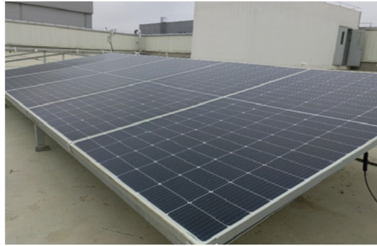
Site of "Lotus" module in Hefei factory
